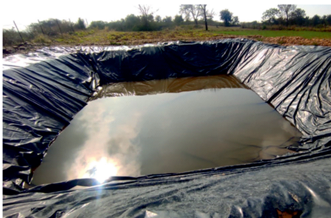
Rainwater harvesting tanks constructed in farmers' fields
