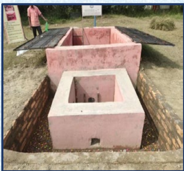
Fig. 7: Overview of drainage cum recharge structure developed at RPCAU, Bihar
