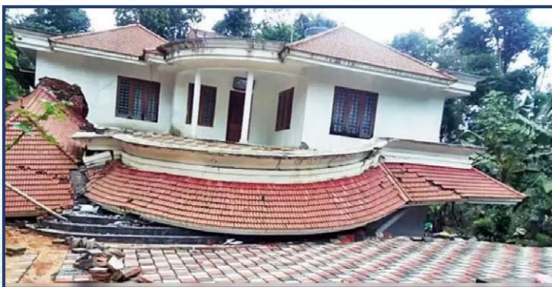
Fig. 3: Damage to building due to sinking of land
